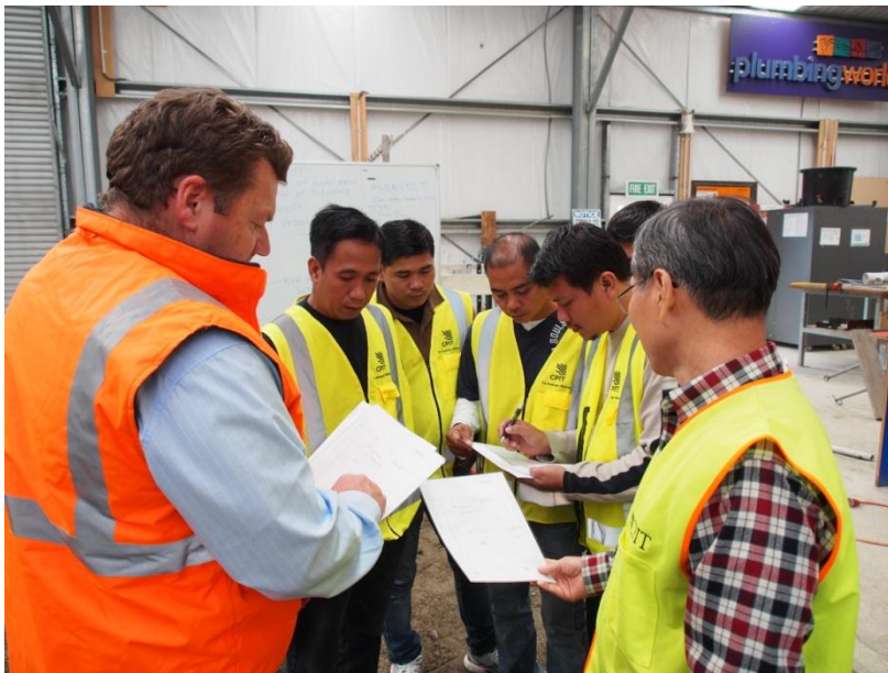
Adrian Couchman from Transfield discusses duct laying plans with new employees at CPIT’s dig training facility.
